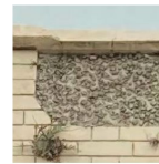
REN-E Render - existing Repaired & painted Location: Existing facade ornamentation
