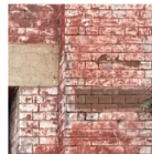
BR-E Brickwork - existing Existing paint stripped Location: Existing facades
