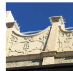
REN-D Render - decorative mould (existing) Repaired & painted Location: 197-199 + 201 facade ornamentation
