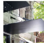
SP Steel Plate Paint Finish Location: Rooftop bar awning
